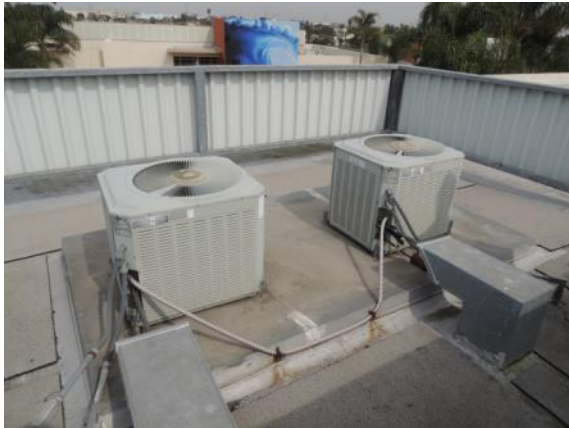
Photo #55: Typical rooftop condensing units
