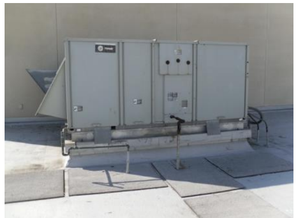
Photo #54: Typical rooftop package AC unit
