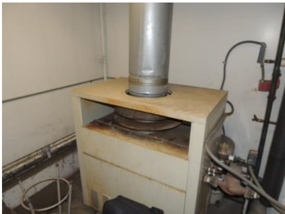
Photo #51: Hot water boiler for locker room showers
