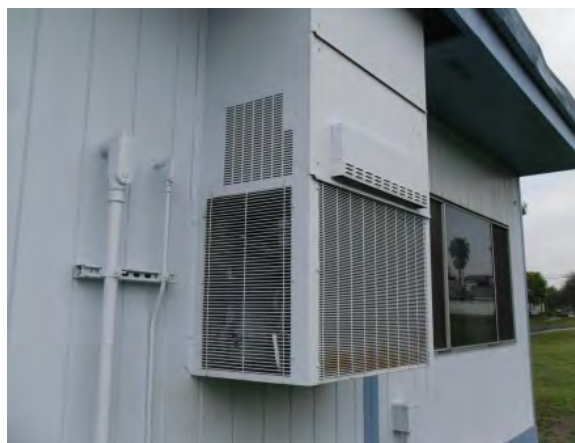
Photo #49: Portable classroom heat pump unit
