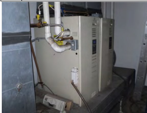
Photo #51: Cafeteria heating gas furnaces
