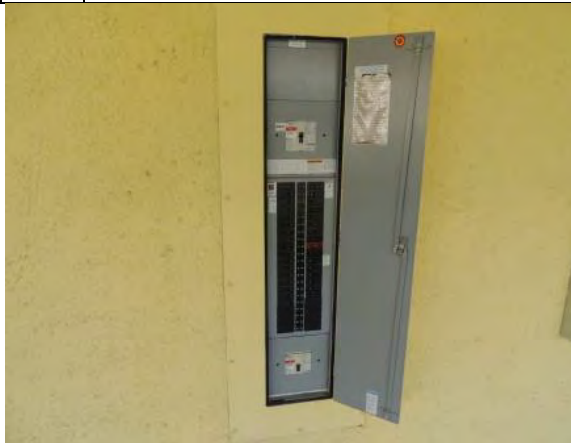
Photo #42: Typical classroom electrical panel
