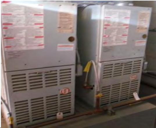
Photo #37: Heating gas furnaces
