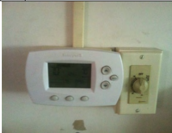
Photo #33: Thermostat and timer in classroom
