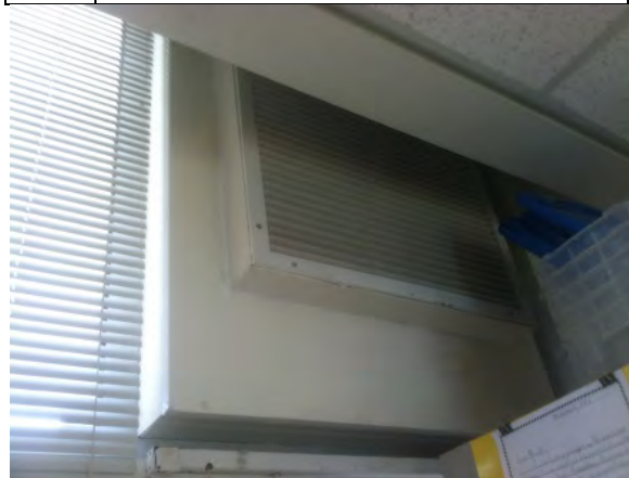
Photo #36: Typical outside air intake louver in classroom
