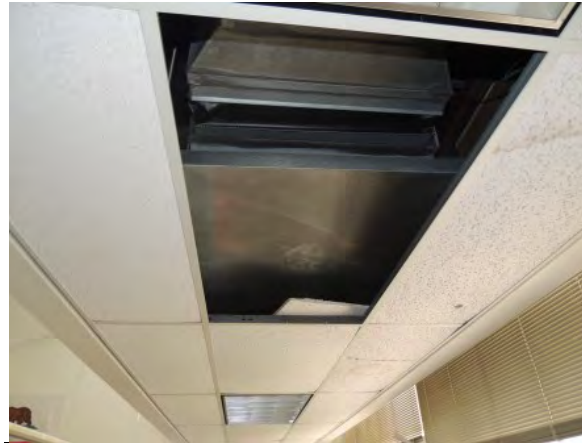
Photo #32: Typical gas furnace in ceiling space
