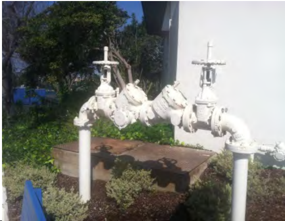
Photo #43: Backflow prevention assembly
