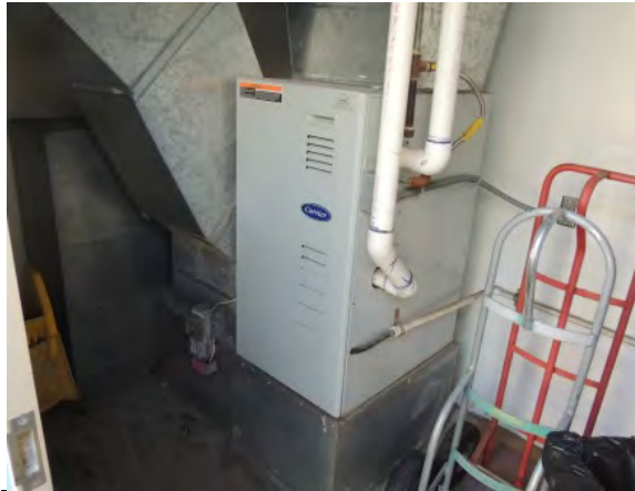
Photo #31: Typical gas furnace in mechanical closet
