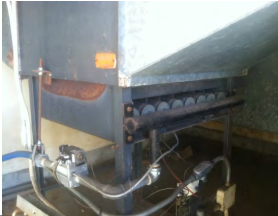
Photo #37: Multipurpose room gas furnace
