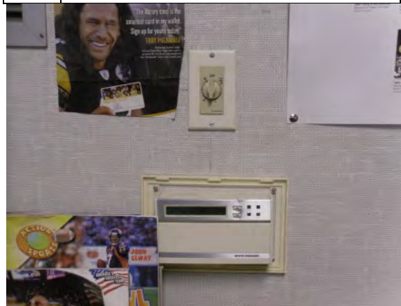
Photo #34: Thermostat and timer in portable classroom
