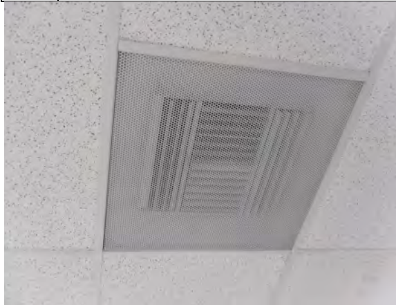
Photo #35: Typical 4-way diffuser
