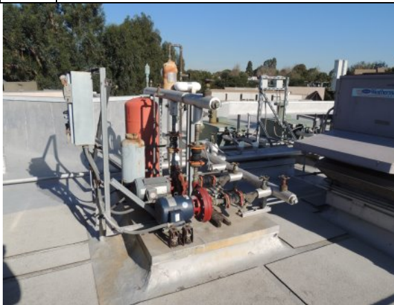
Photo #35: Heating water pumps
