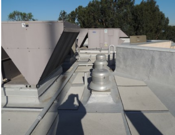
Photo #37: Bathroom exhaust fans
