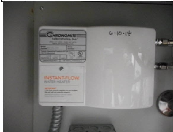
Photo #46: Typical "Instant-Flow" water heater
