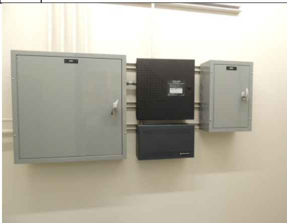
Photo #47: Fire alarm panels
