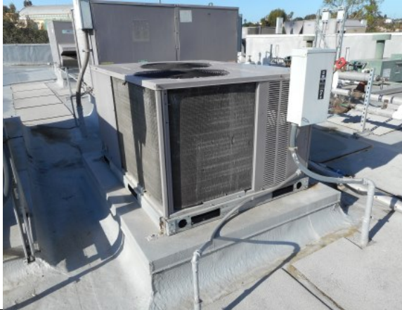
Photo #31: Packaged air conditioner unit
