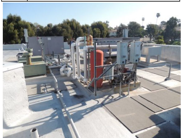
Photo #36: Heating water pump disconnect switches and expansion tank
