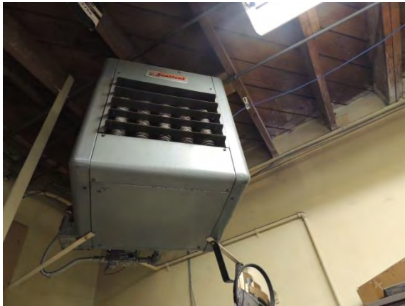
Photo #15: Typical ceiling gas unit heater
