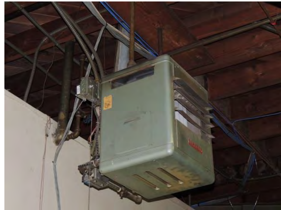
Photo #16: Typical ceiling gas unit heater
