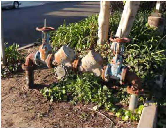
Photo #55: Backflow prevention assembly
