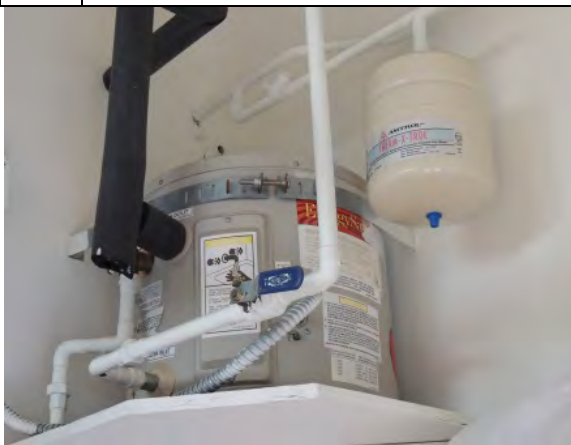
Photo #53: Typical janitor closet water heater
