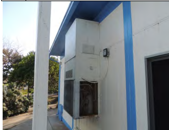
Photo #48: Typical portable classroom heat pump unit
