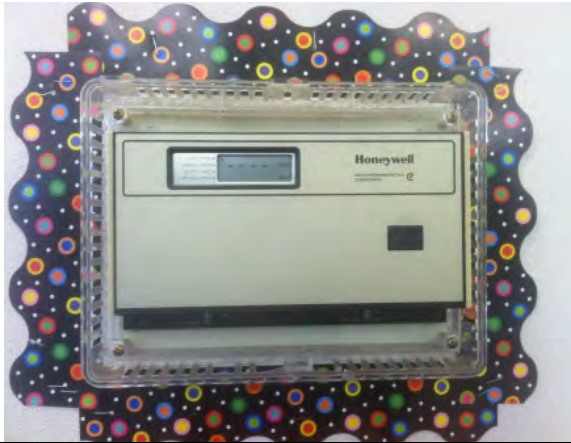
Photo #49: Typical portable classroom thermostat
