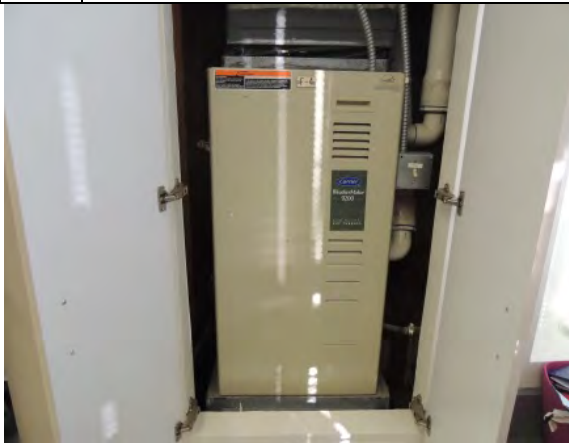
Photo #47: Gas furnace in health office
