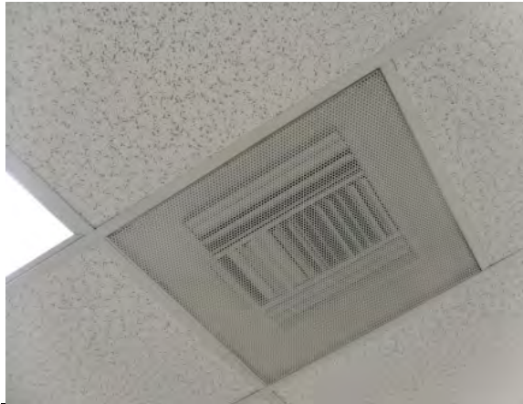
Photo #49: Portable classroom 4-way diffuser
