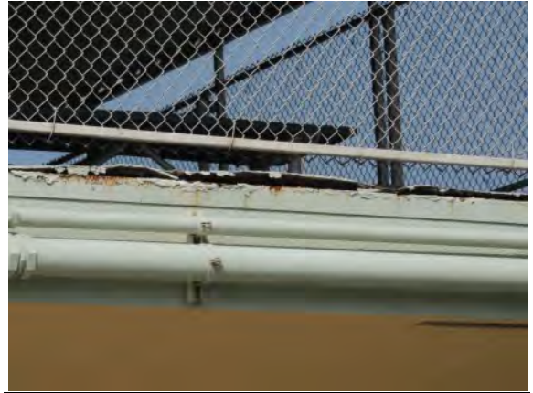
Photo #14: Deteriorating decking edge
