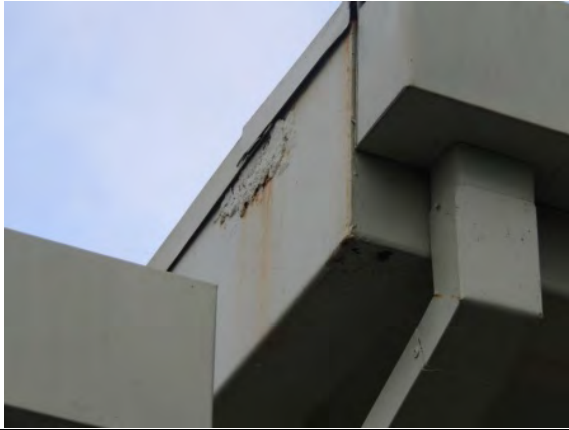
Photo #25: Gutter and flashing
