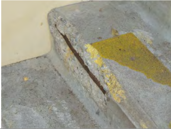
Photo #13: Deteriorating steps
