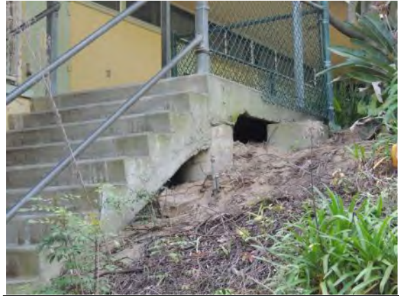
Photo #8: Area where dirt has been washed out under stair system
