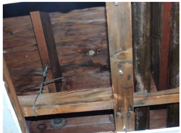
Photo #24: Ongoing classroom roof leak
