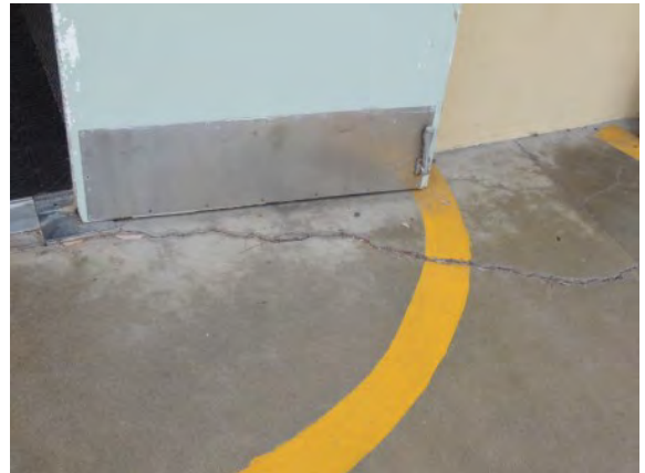
Photo #16: Deteriorating floor slab
