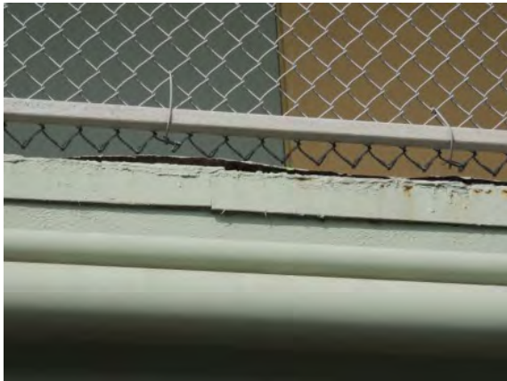
Photo #15: Deteriorating decking edge
