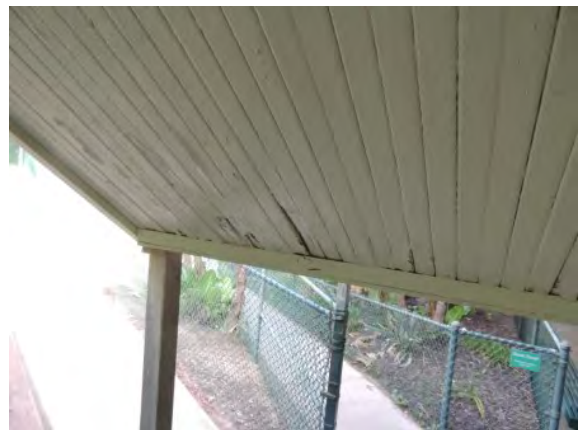
Photo #12: Deteriorating covered walkway
