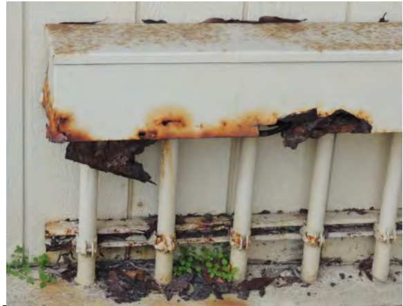
Photo #56: Deterioration at exterior electrical enclosure
