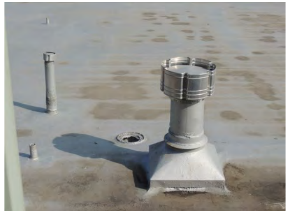
Photo #18: Missing roof drain cover
