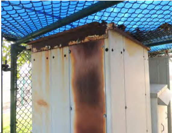
Photo #55: Deterioration at electrical panel enclosure
