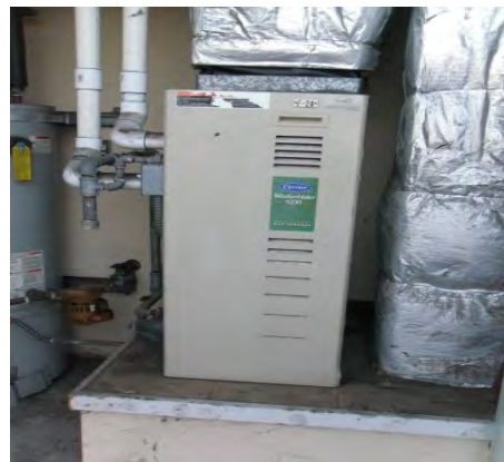
Photo #46: Gas furnace in mechanical closet
