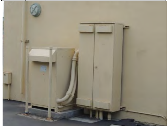
Photo #52: Transformer and electrical panels
