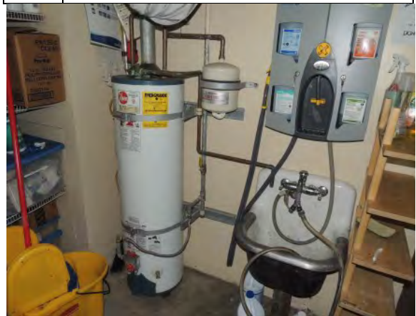
Photo #64: Typical water heater
