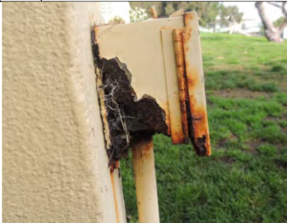
Photo #57: Deterioration at exterior receptacle enclosure
