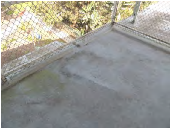
Photo #17: Deteriorating floor slab
