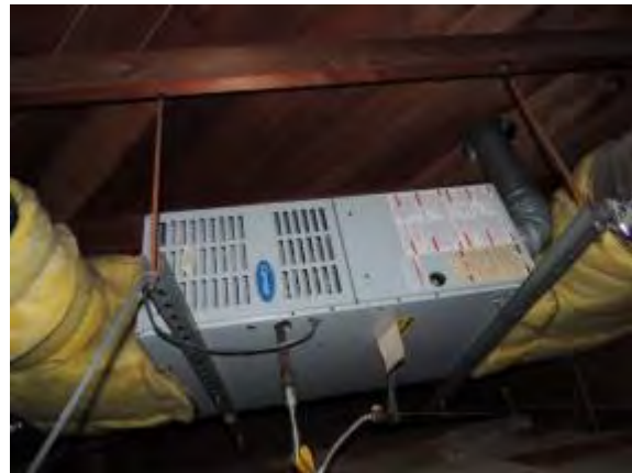
Photo #34: Typical ceiling mounted gas-fired furnace
