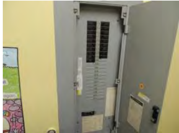
Photo #40: Typical classroom electrical panel
